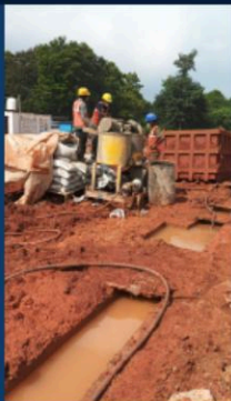
ACTIVE GEOTECHNICAL SITE WORKS
